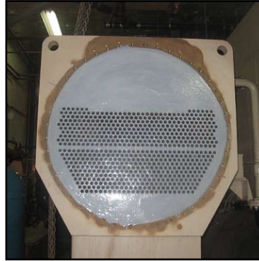
Tube sheet completed.
