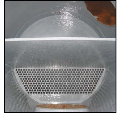
Water box completed.
