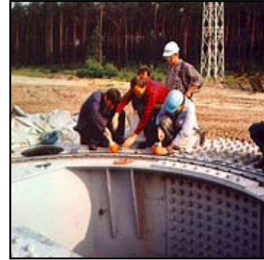
A team of applicators was required to apply all the Belzona® 1111 quickly, to allow time for the rings to be located
