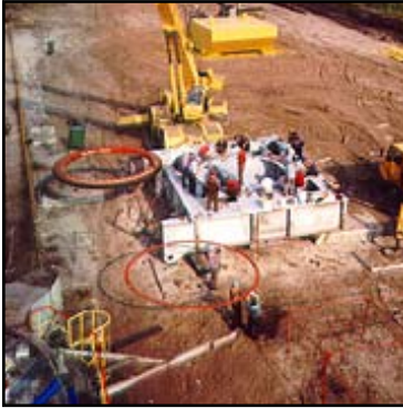
General view of the excavator partially dismantled for maintenance
